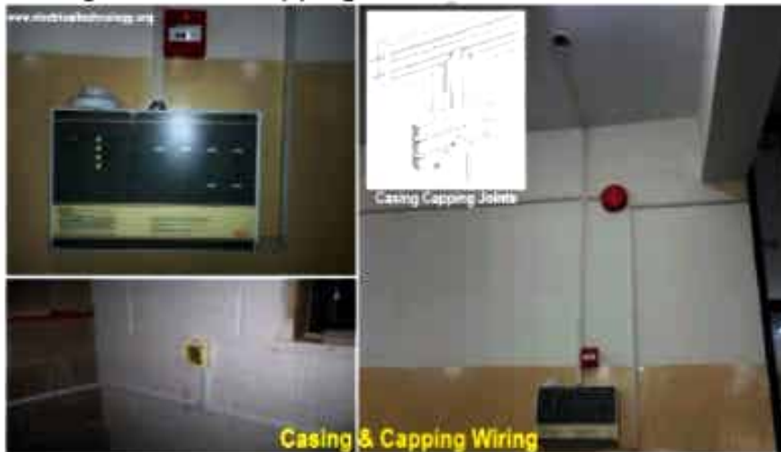
(Fig.5.2. Casing & Capping Wiring)
